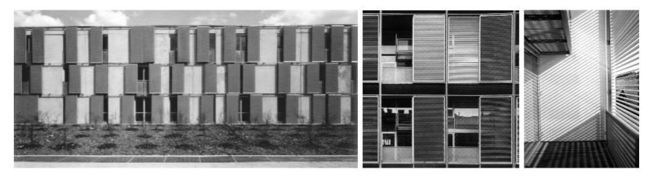
The living spaces should open to a protected space, sometimes an outside terrace or sometimes a "jardin d'hiver". By using the cavity between two skins of the building, opening panels could give the opportunity to control and modify the air, the light, the cold, the outside view.
